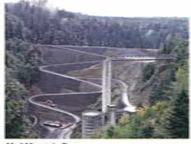
Mud Mountain Dam
